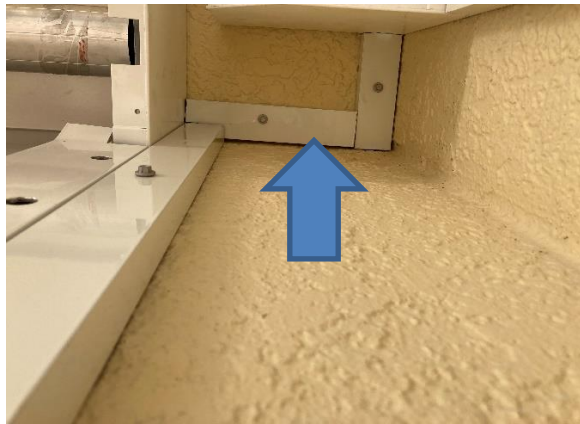
View looking up at ceiling showing u-channel connecting 2 assemblies
